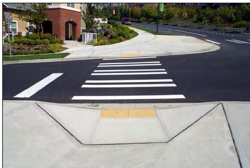
Curbs must be ADA compliant
