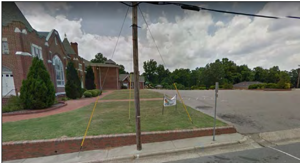
Some sidewalks in Carthage are obstructed and require ADA accessibility improvements. This utility pole and street sign adjacent to First Presbyterian Church on South Ray Street are examples of barriers to pedestrians in wheelchairs.
