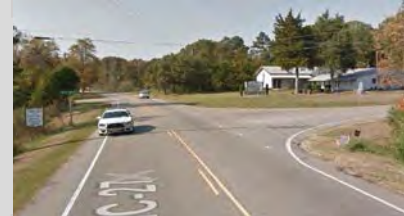
McReynolds Street Leaving Courthouse Source: Google
